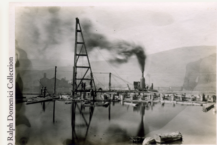
Driving log piles to the bedrock during the Age of Steam
