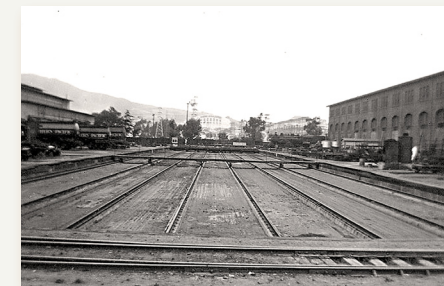
The locomotive back shops (left) and car shops (right) were located just to the north of the Roundhouse. Straight ahead, due west is the Cow Palace arena. The back shops were behind the Roundhouse and handled heavy repairs. In the center are the transfer pit and transfer table for moving cars and locomotives from one stall to another.
